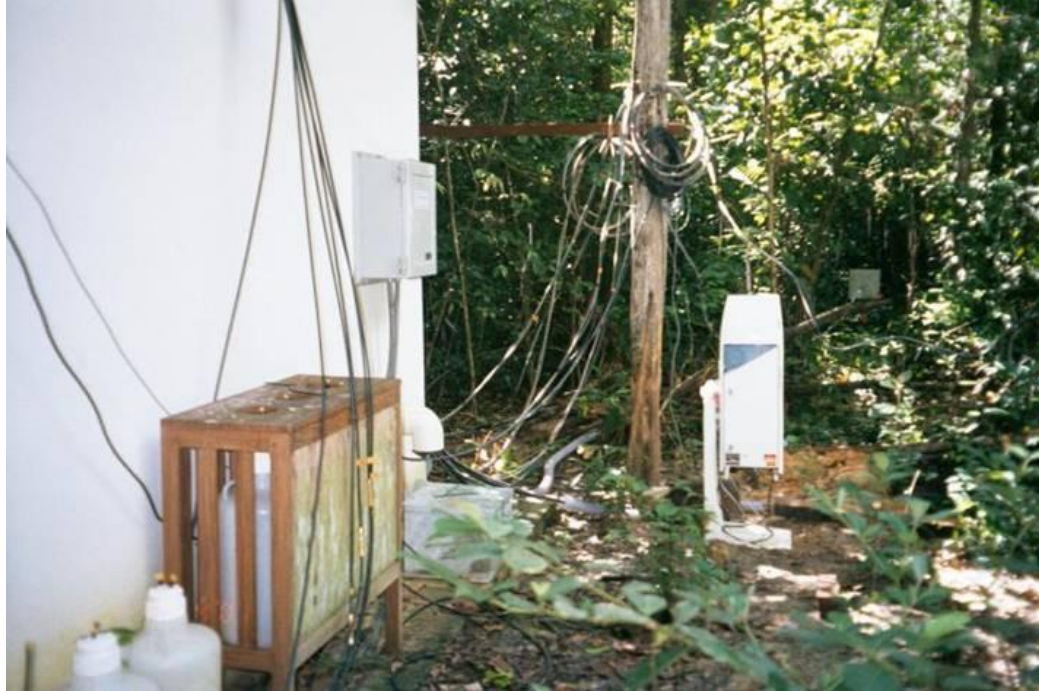
Vaisala CT-25K ceilometer as installed at the old-growth forest site located at the km 67 Eddy Flux Tower site in the Tapajos National Forest.
