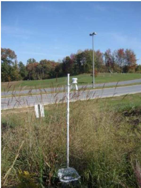
Figure 3. Data logger mounted at the rain garden location on GSFC campus.
