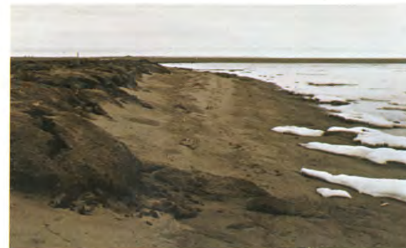
Figure 67. Coastal beach with slumping peat mat. Vegetation on the peat has been killed by salt. Height of the bluff is about 1 m.
